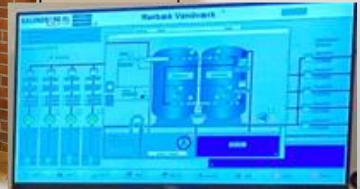
Nyt SCADA Supervisory control and data acquisition
